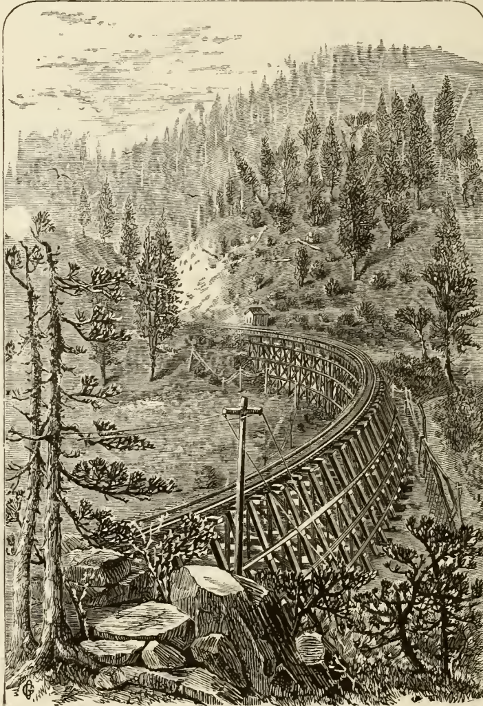
SECRET TOWN, TRESTLE WORK.
